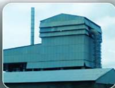
WASTE WATER PLANT CAPACITY 10 KL PER HOUR
