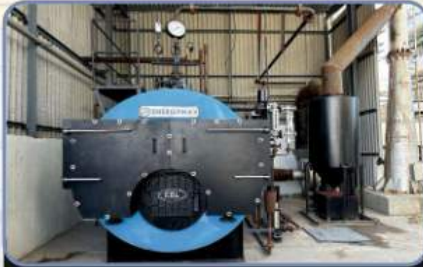
TURBOMAX (Solid Fuel Fired Package Steam Boiler.)
